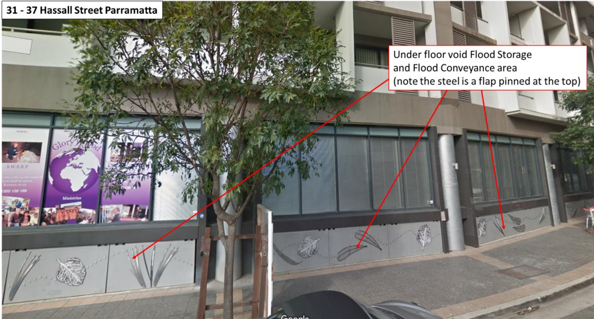
Plate 8 Example of under floor void flood storage and conveyance (31 - 37 Hassall St Parramatta)
