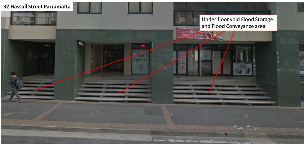
Plate 7 Example of under floor void flood storage and conveyance (32 Hassall St Parramatta)
